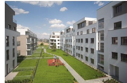
Ostoja-Wilanów (stage 4). Date of delivery: 2009 No. of units: 228 apartments (22,336 sq. m).
